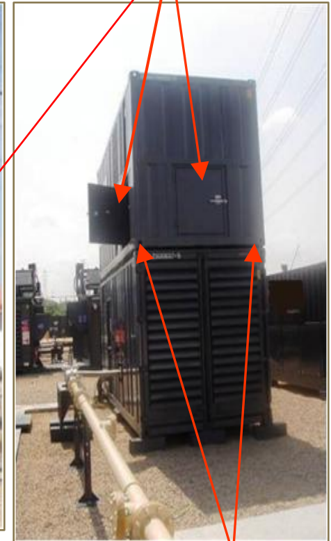
Standard twist locks used to connect containers together
